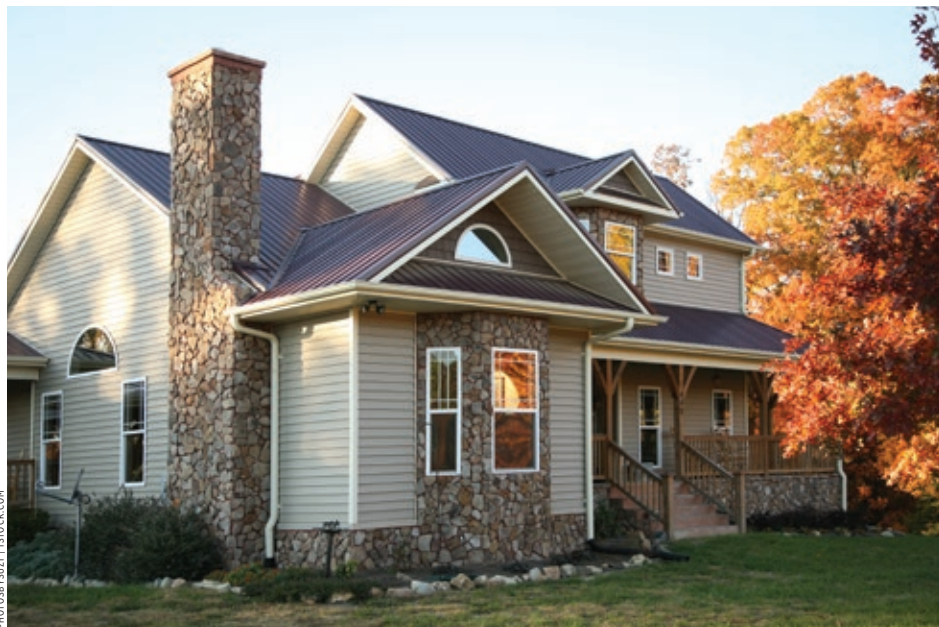
Metal roofing is more expensive, but the energy savings and fire-resistant qualities make it worth the investment.
