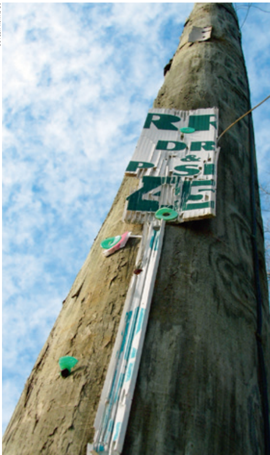
Signs and objects illegally attached to utility poles can be a safety hazard for line crews that climb these poles.
