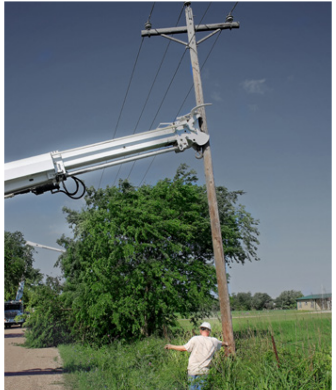
Crews lined the streets to reset numerous downed poles.
