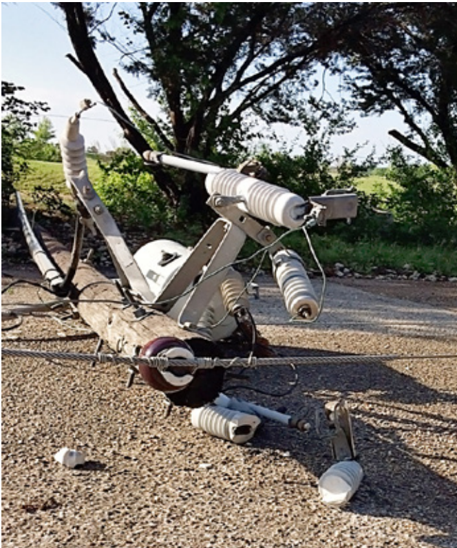
Linemen faced challenges such as this downed electric pole throughout a majority of HILCO Electric's service area.
