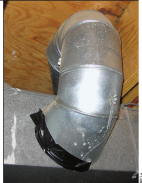
Despite how appropriate its name sounds, duct tape is not a good choice for sealing duct work.
